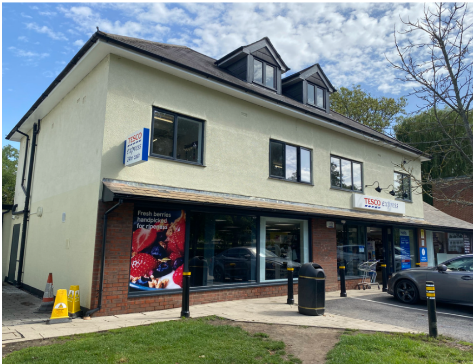
Photos of the sign installed
